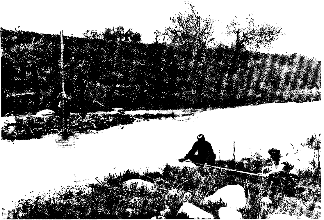
Surveyors at work, 1928 (Tsentral'nyi Gosudarstvennyi Arkhiv Kinofotodokumentov i Zvukhosapisei Respubliki Kazakhstana—or TsGAKiZ RK—Turksib Collection, 8-2215).
